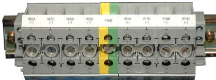
Figure 1-63 Input terminals of the I-type DC PDU
